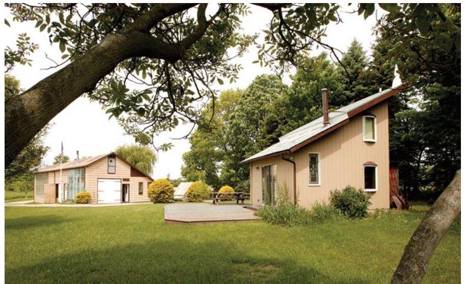
The Little House. Wilson’s home and shop were all in one in The Little House (right) before he built The Home Shop (left).
